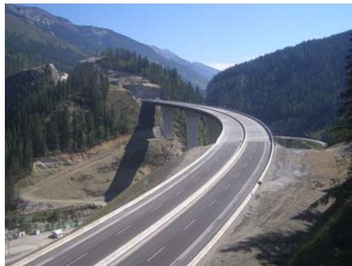
Park Bridge east of Golden, British Columbia
