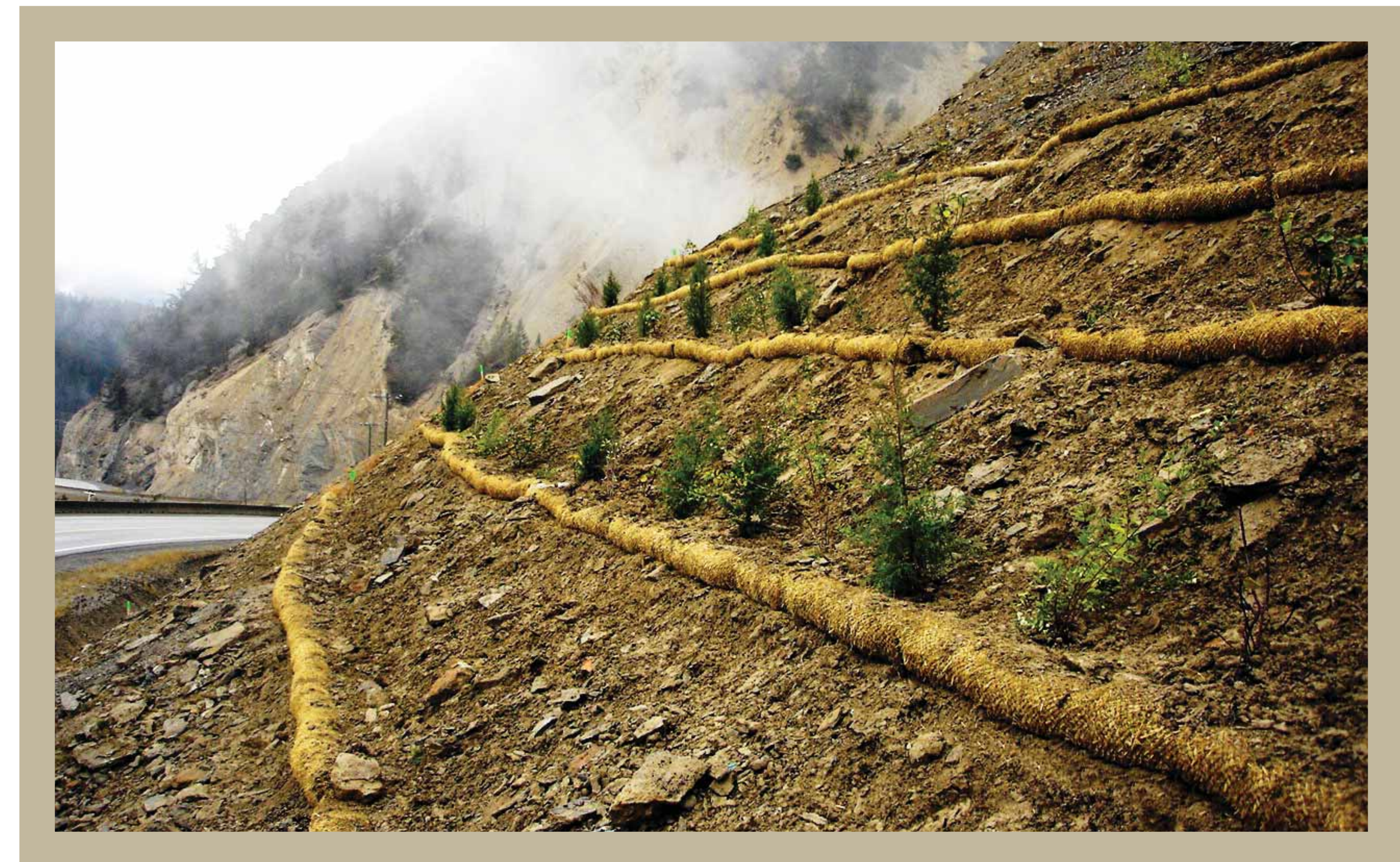
Straw “log” terraces are created to encourage moisture retention and improve surface soil stability while plantings of native vegetation become established.
