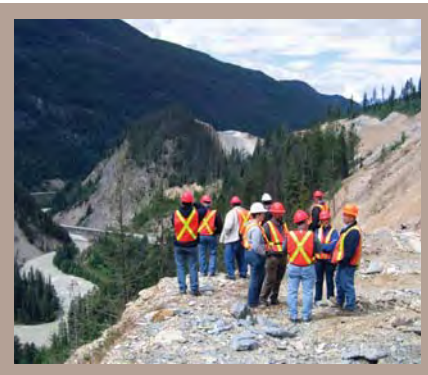
Community liaison committee inspects progress in June 2006
