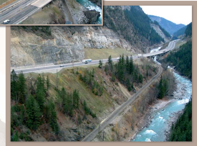
Completed Yoho Bridge
