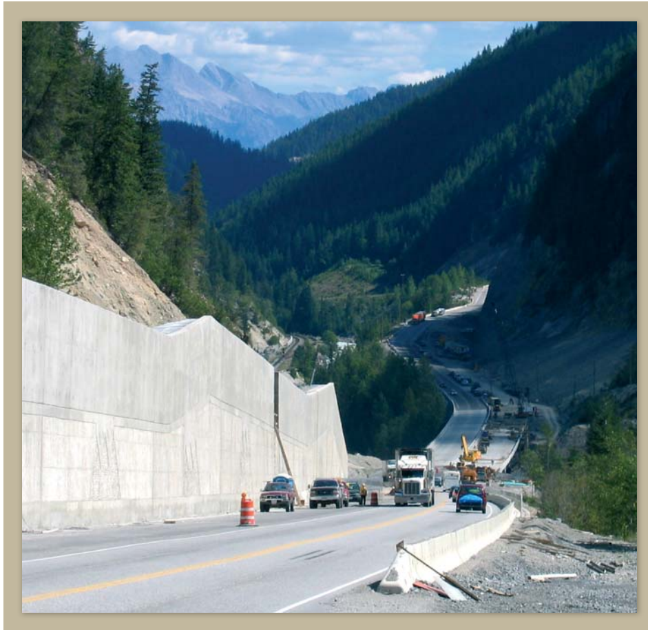
Yoho Bridge under construction, August 2004
